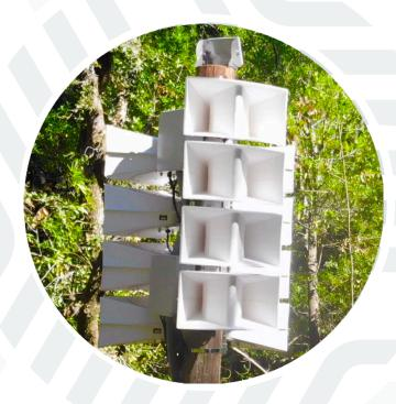
Mill Valley community leaders decided that the city's outdated mechanical air raid sirens needed to be replaced with modern emergency warning system installations that continue to operate when existing power and communication infrastructure goes down.
