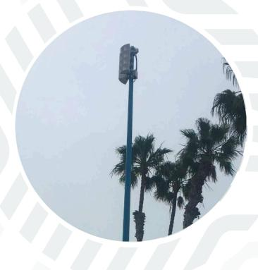
Shortly thereafter, the City of Newport Beach installed mechanical tsunami warning air raid sirens. In 2019, city officials found that the metal sirens had rusted and were non-functional. City staff determined it was more cost effective to replace the air raid sirens with non-mechanical systems that included voice broadcast capabilities.
